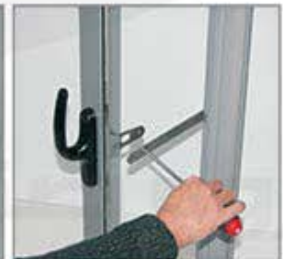
Vent disengaged from limit stop
